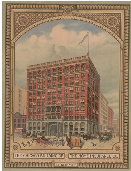
Figure 1: Home Insurance Building (1885), Chicago. Source: Library of Congress .
